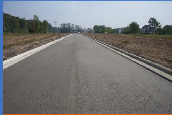
Roller Compacted Concrete Pavement
