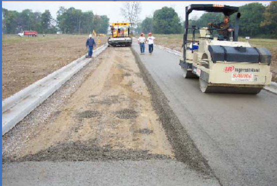
Roller Compacted Concrete Pavement
