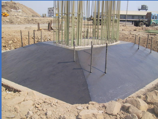
Pile Cap – Bandra Worli Sea Link Project
