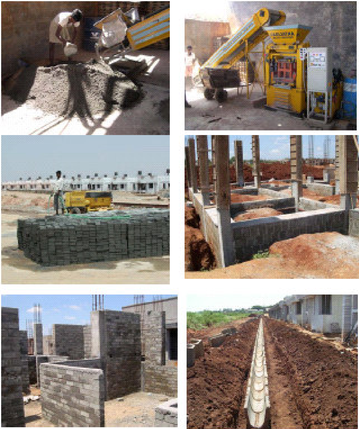
Fig 2. A&B: Dry concrete and machinery used in the manufacture of bricks and paving blocks. C: Curing of the concrete paving blocks. D: Large concrete blocks for housing foundation. E&F: Concrete bricks (E) and gutters (F).
